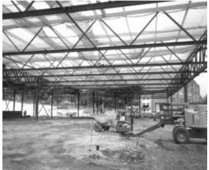
Safety nets installed prior to sheeting. Note the net is fixed as close to the underside of the roof as possible to minimise the extent of any fall
