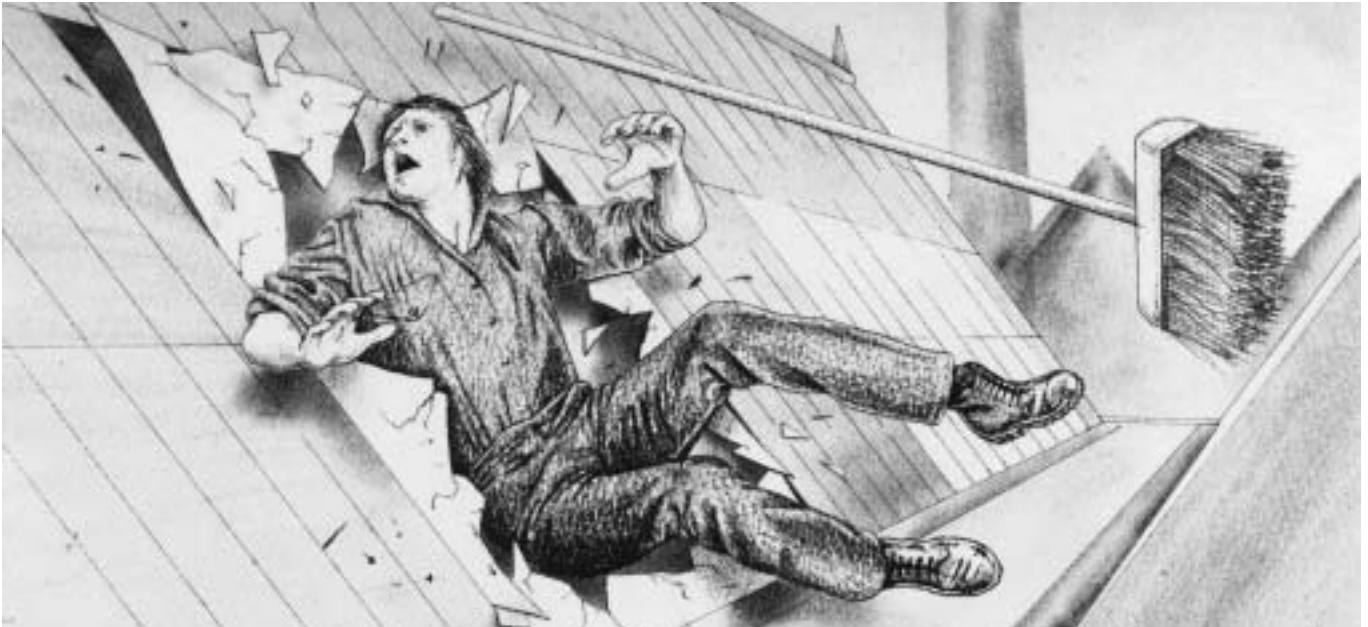
A man cleaning valley gutters on an asbestos cement sheet roof stumbled and fell to his death
