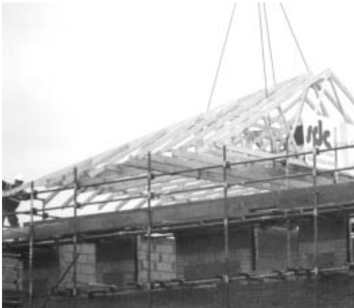
Roof truss built on ground and lifted into position avoiding the need to work over open joisting later on
