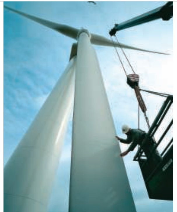
Reaching new heights in wind turbine blade production.
